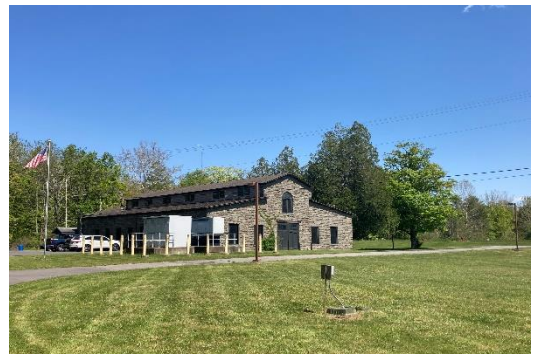
Edmund T. Cloonan Water Treatment Plant
