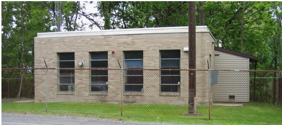
Golden Hill Pump Station
